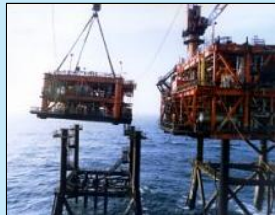
Figure 2 Structural Removal of Oil and Gas Platform Decommissioning
