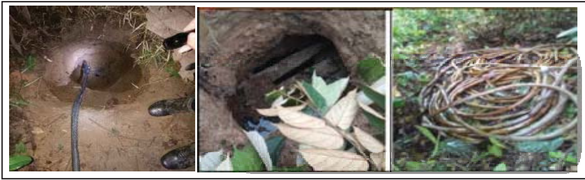
Figure 2 Illegal tapping on hidden area.
