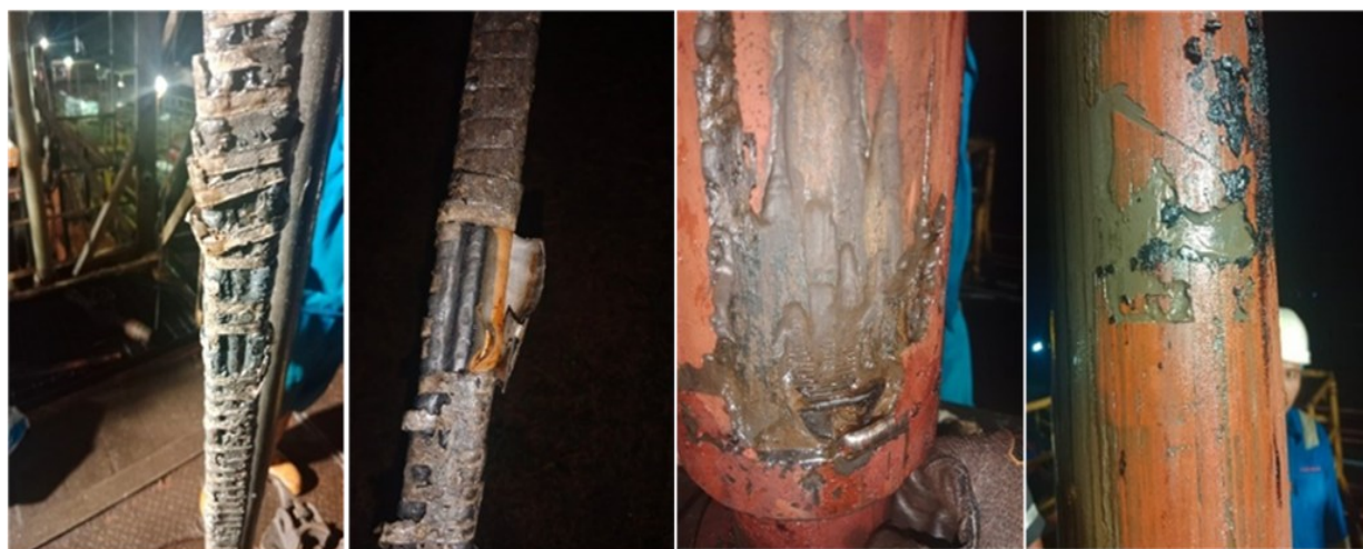
Figure 1. Damage on the ESP cable and bottom hole assembly of the D-04 well
