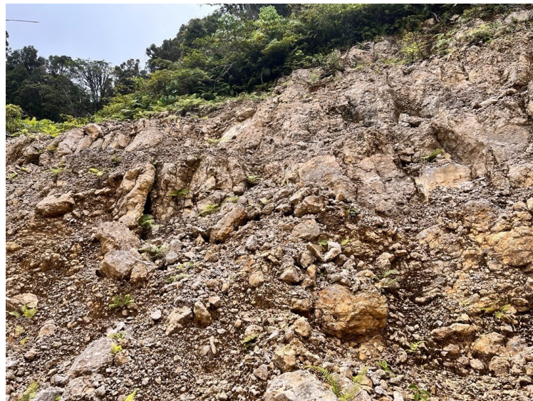
Figure 21. Highly faulted Miocene outcrops were observed at Iono Besar. Outcrops of Faunai Formation were not accessible. However, it is likely that Faunai Formation exhibits similar characteristics of extensive faulting. (Photo by Nauw 2025).
