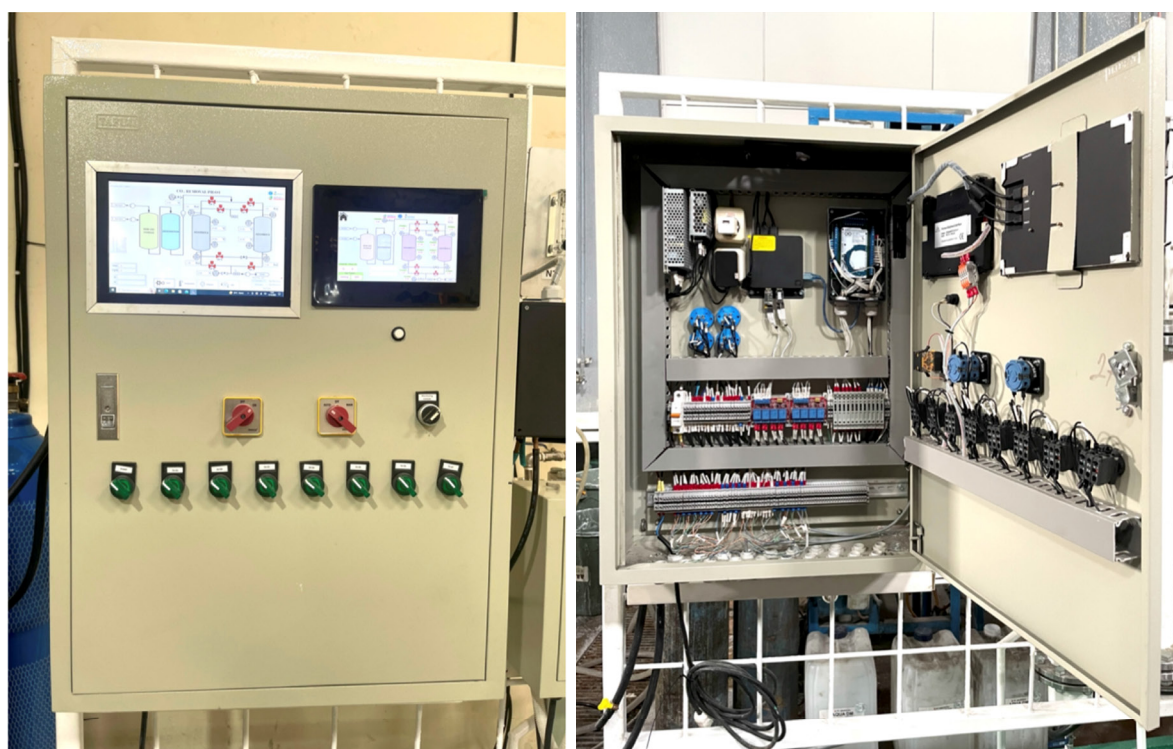
Figure 10. (a). Control panels equipped with LCD-HMI, (b) instrumentation equipped with online CO 2 Analyzer
